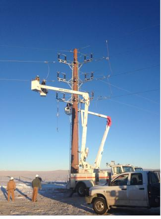
The pictures above show our NEA line crew working together with the contractor, Mid Plains Power, making the final connections on the switch structure just north of Lusk, near the intersection of Hwy 85 and Kirtley Road. This was the final major step in getting the new substation ready for service for the ONEOK pump station.
