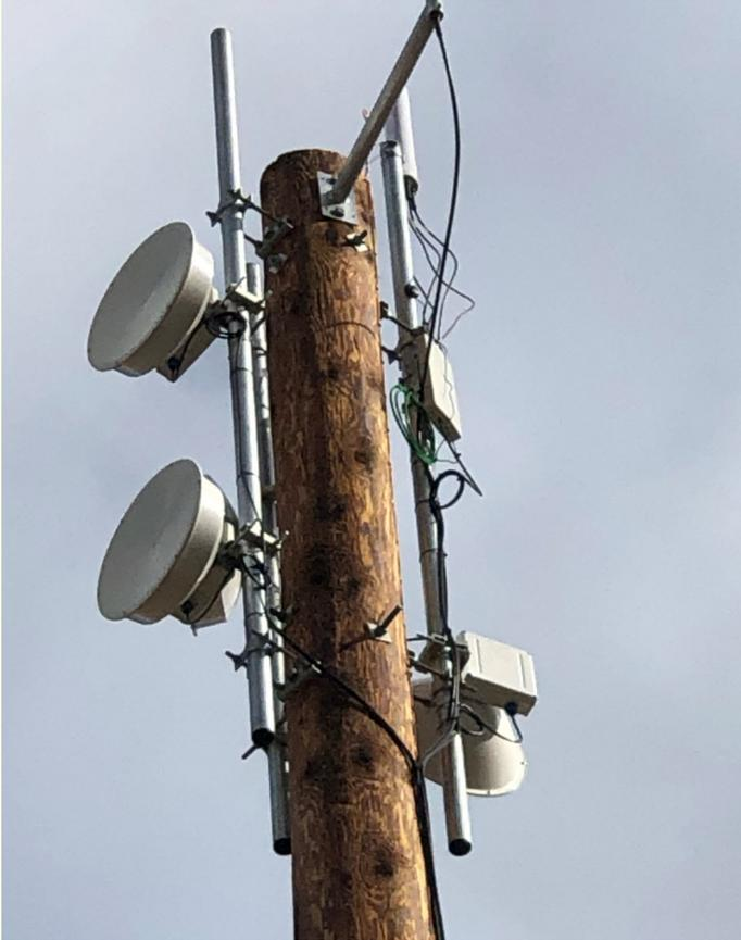
Photos Left: A collector box, which holds meter readings, hangs on the side of this pole and from the meter running up the pole is an antenna that rises a few feet above the 65ft pole. At the top, sharing space on the pole, Vistabeam's equipment supplying internet to the area and sending our meter signals to a Landis & Gyr service center in Kansas.
